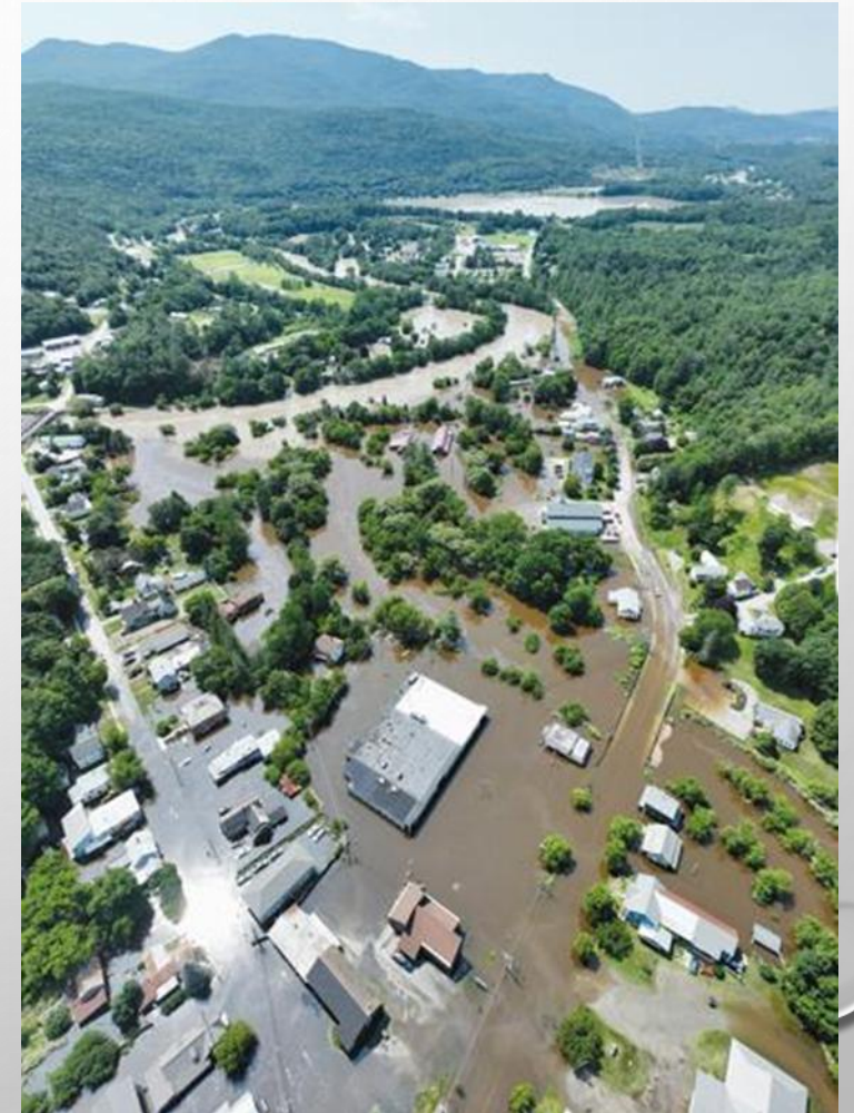
July 2023 Flood, Johnson Village
