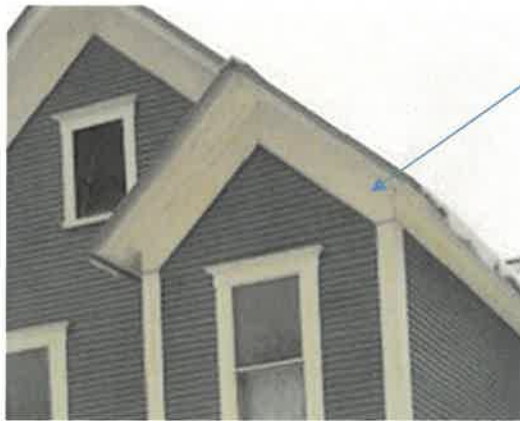
Frieze intersection at corner board example at 68 George Street
