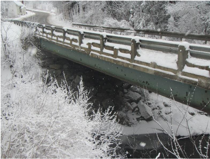
Photo 1 - South Elevation of Bridge
