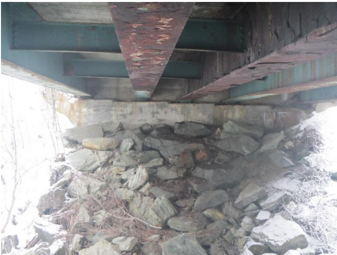
Photo 3 - Abutment No. 2 Elevation
