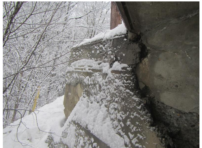
Photo 12 - Typical wingwall repair
