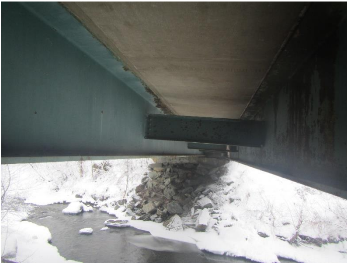
Photo 9 - Girder Nos. 4 and 5, looking west
