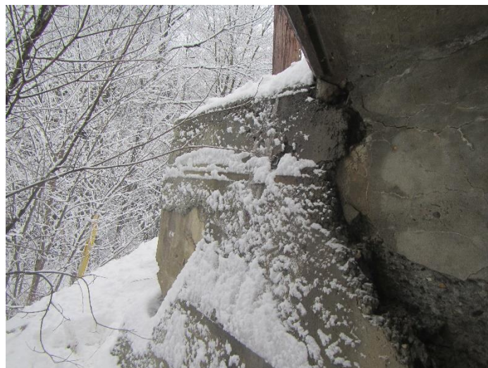
Photo 12 - Typical wingwall repair
