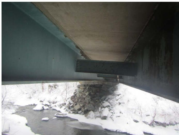
Photo 9 - Girder Nos. 4 and 5, looking west
